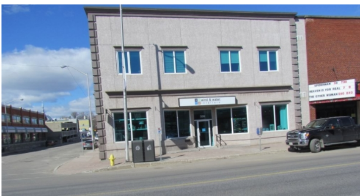
326 2nd St. S. Palace Theater -Bergman & Nelson-Bergman Building
